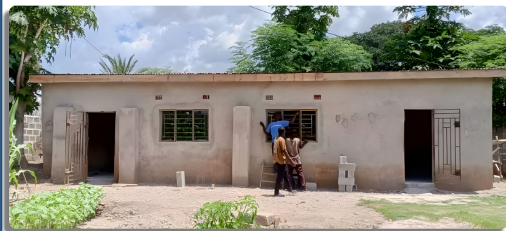
New Church Building in Ndola
