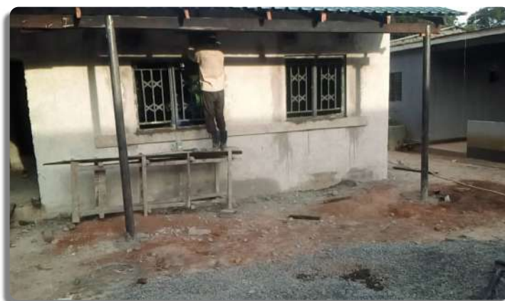
Plastering the Walls
